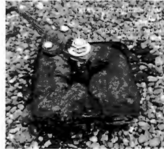
Pitch Pan: Pitch pan fractured allowing water into the building directly.
