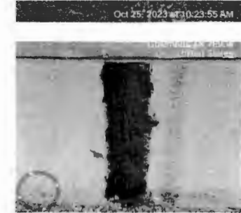
Flashings UV unstable allowing rapid decay.
