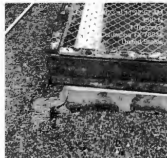
Jail Yard covering severely rusted.
