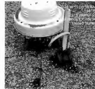
Heavy patching observed around the air vents.
